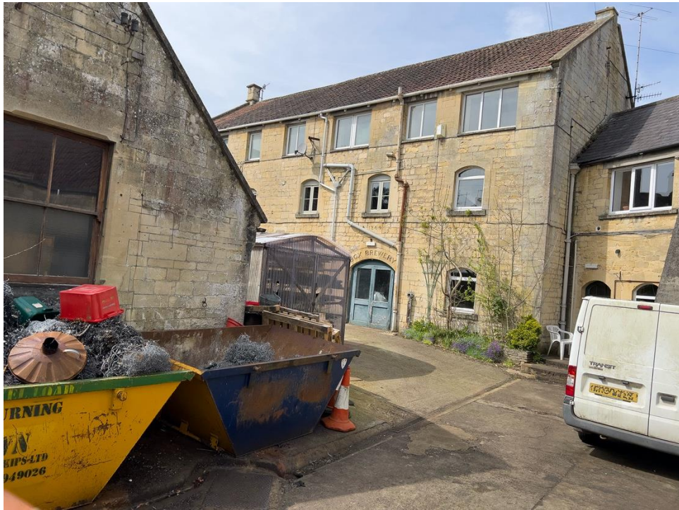
Main brewery building, with datestone over entrance
