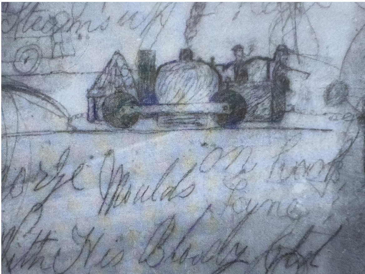
Graffiti within Clift quarry includes this representation of the underground steam locomotive. An account in The British Architect of 1883 (vol 19, p143) states that "Without exception, we do not think we have seen a more thoroughly ugly bit of machinery than the steam infant Hercules, which is to convey us into the interior of the hill before us" (photo D. Pollard)
